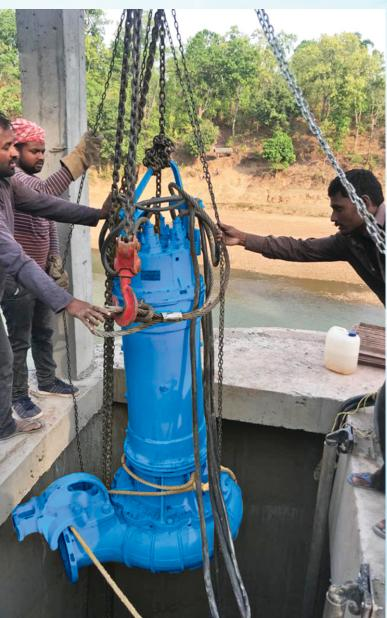
2nd stage PS was constructed with VT pumps which have lighter duty as they are relieved of level fluctuations & face less silty water, as compared to Submerged Centrifugal Pumpsets in 1st stage
