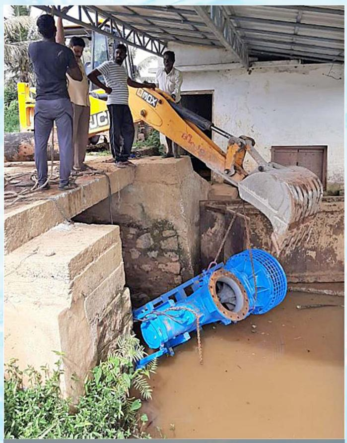
Submerged Elbow pumpsets are Fully Portable & hence easily Installable
