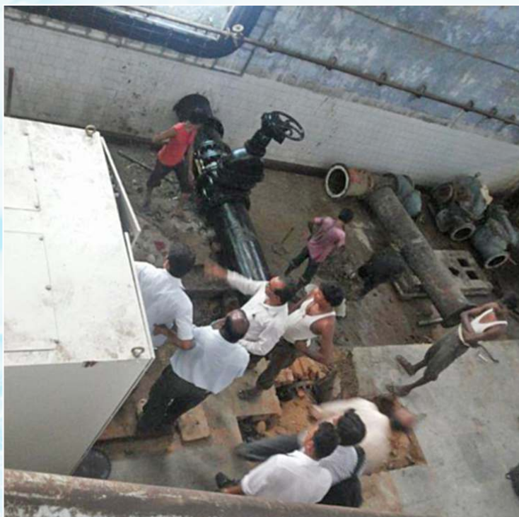
Replacing Dry installed HS CF pumpsets by Wet installed Submerged CF pumpsets; utilizing Old Suction pipes as New Delivery pipes
