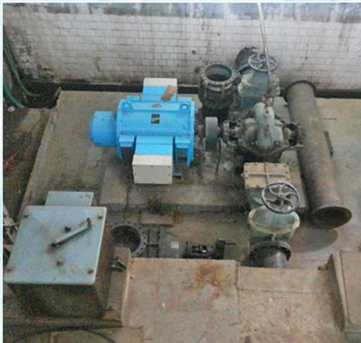
Augmentation of existing Dry Installed HSCF Pump based Water Pumping Station without disturbing Civil Structure & Grouted Suction Manifold.
