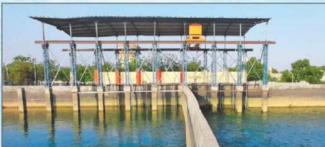
Gujarat Water Grid 300mld Sadulka DBC Offtake (SCF Pumpsets Installed Vertically on Auto-Coupling)
