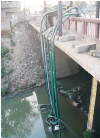
Being used to pump sewage from an open drain & incoming grit chamber.
