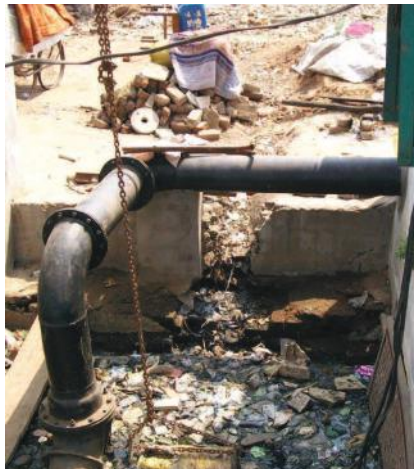
Being used to pump sewage from an open drain & incoming grit chamber.
