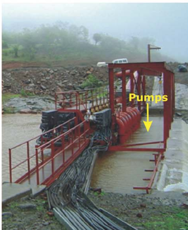
Aqua's pumps (270hp) harvest 6000 m 3 /hr of rain water for a pumped storage scheme
