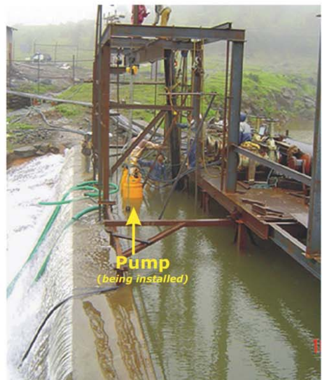
Aqua's pumps (270hp) harvest 6000 m 3 /hr of rain water for a pumped storage scheme
